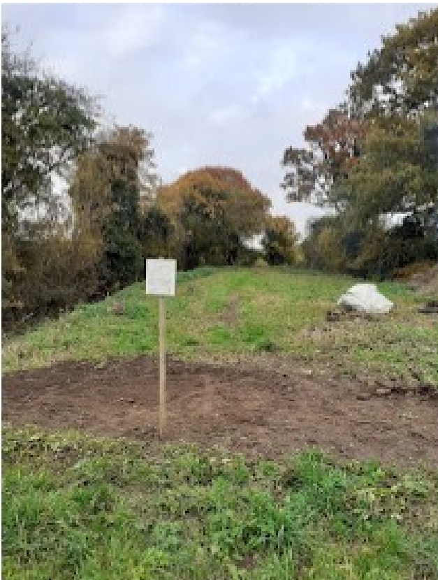
Creating a new access slope
